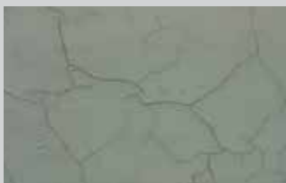
Concrete with Ordinary Cement
